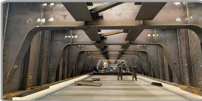
Thailand Railway Bridge-20M
